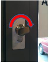
Unlock the door by turning the turnkey lock in the centre of the door clockwise until the latch is released.
