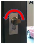
Lock the door by turning the turn-key lock on the centre of the door anticlockwise until the catch is home.
