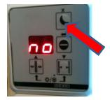
On the automatic doors and press the top button. If the doors are open the key tab display will show 'No' and the doors will then slide shut.
